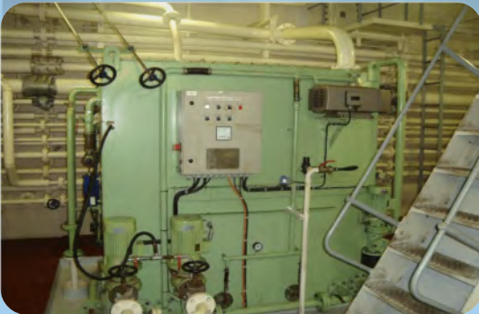
Sewage treatment plant on board a ship.
